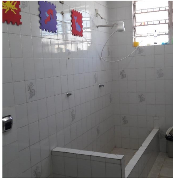
Safe shower facilities – no more exposed wires!
